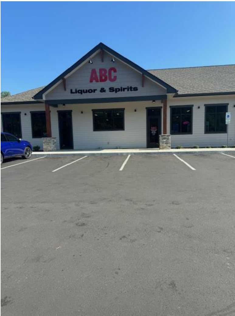
752 W US-19 Bypass, Burnsville, NC.
