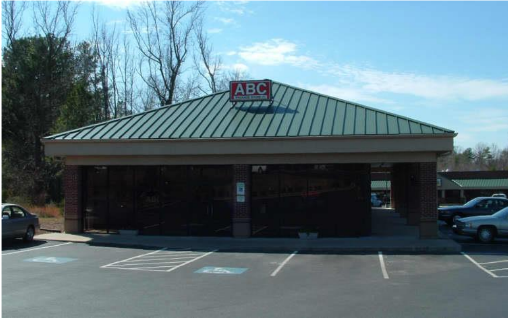
2280 Jefferson Davis Highway, Sanford, NC.
