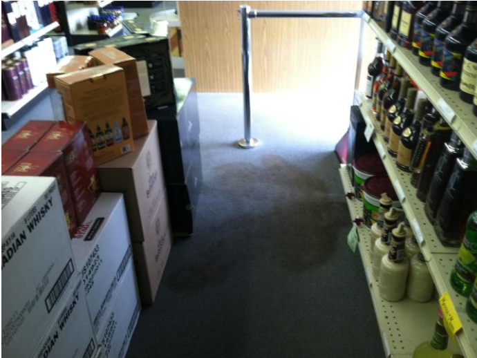
Stains on the carpet at Store 1
