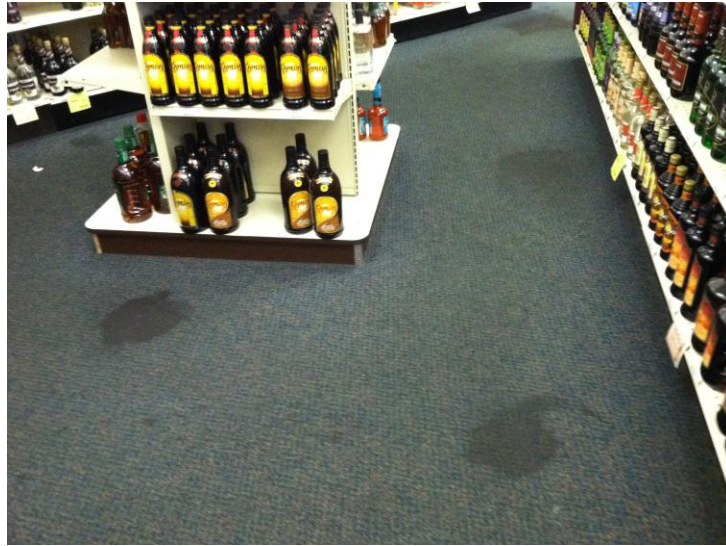
Carpet stains at the Memorial Drive location.
