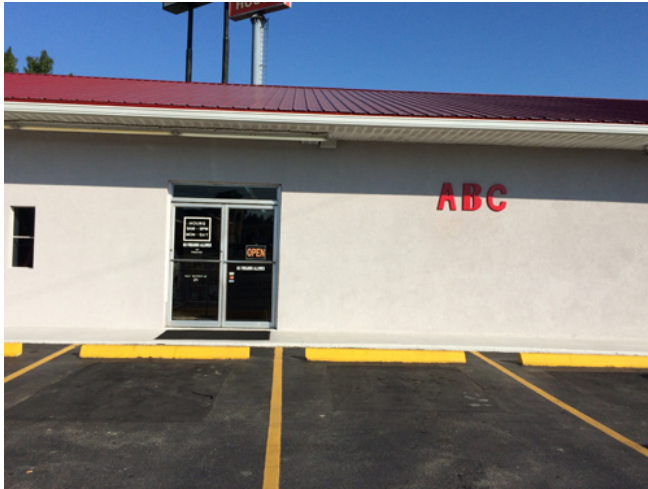
Exterior view after initial audit fieldwork
