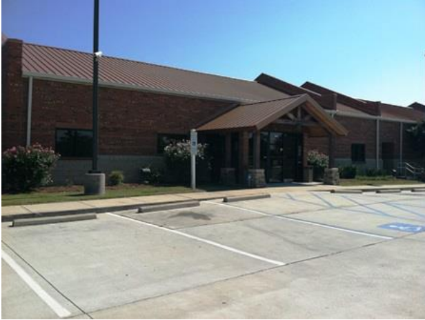
Main office complex in Grandy, NC
