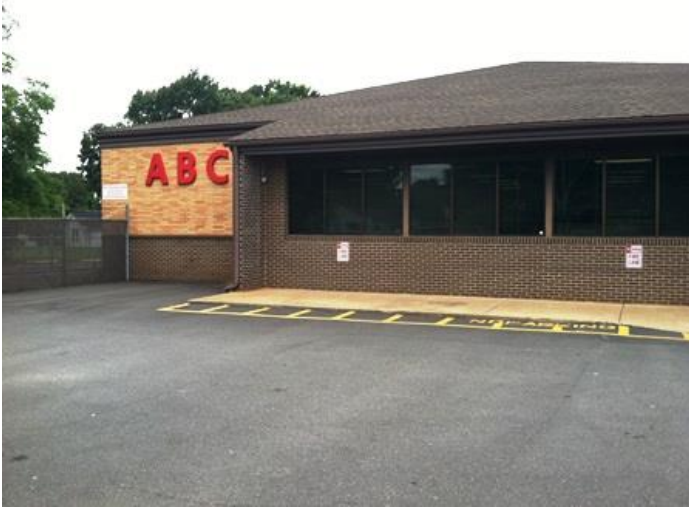
Exterior view of Warren Rd.
